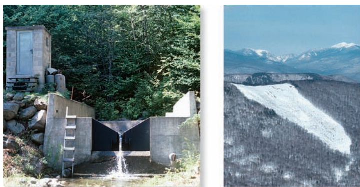
(a) Hubbard Brook dam and weir
